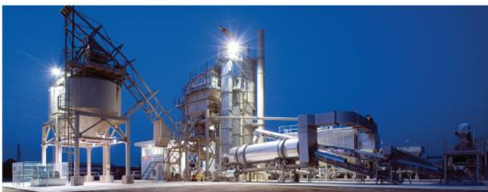
Stationary Asphalt Plant
